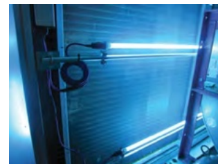
Blue-Tube XL Coil Mount Installation
